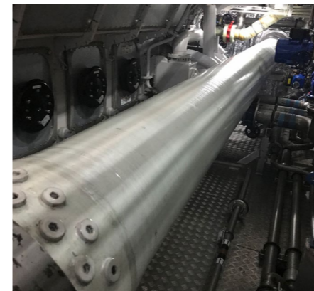
Jaure carbon shaft after installation
