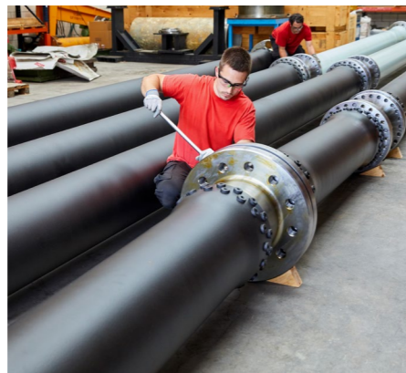
Assembly job at our workshop
