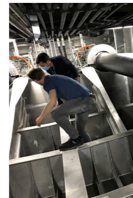
Supervision of installation
